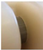
Figure 24 – New corner mount moulded by Tinby A/S showing final design where PUR 1150 Solid is moulded around a Ø30mm ECR fiberglass rod for optimal load transfer
