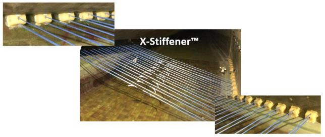
Figure 32 – Final installation of the X-Stiffener™ in the 7MW Levenmouth turbine
