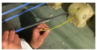
Figure 86 - Photo showing the threading of the rope through corner mount procedure
