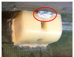
Figure 85 – Photo showing the 60 to 80-degree bracket installed in the PS/TE corner, being held in position by very fast curing SikaForce 7800 BLUE while primary adhesive is curing
