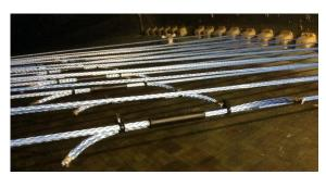
Figure 87 - Photo showing the rope tensioning and locking procedure
